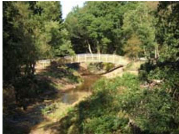
The completed bridge at Hawnby.
