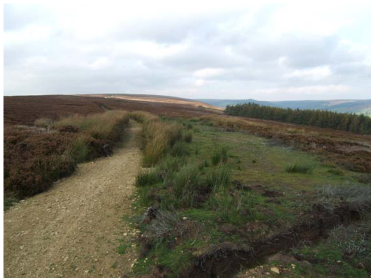
Restoration work on Pockley Moor
