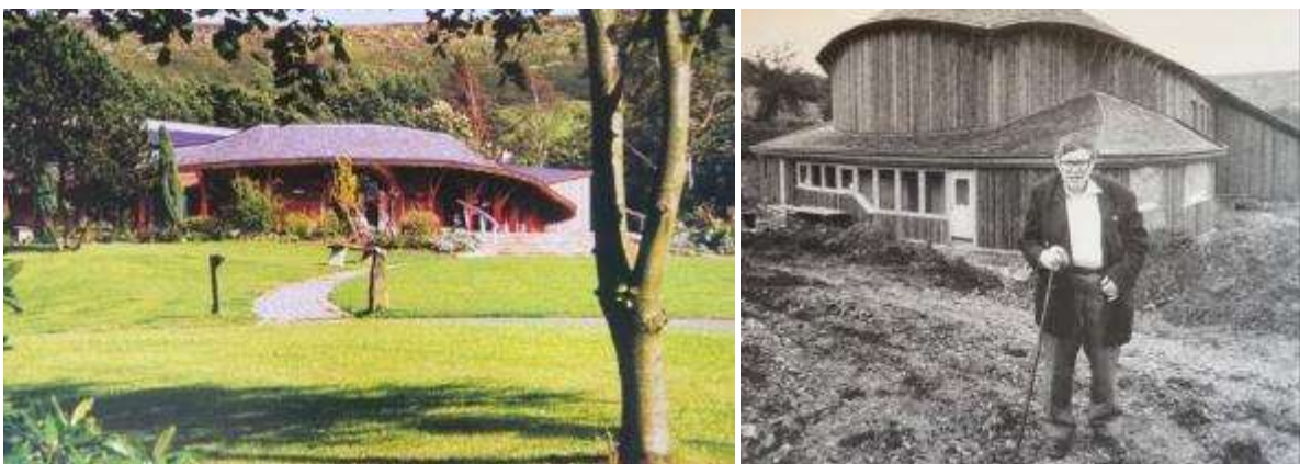
The remodelled Community Centre and the Chapel 1998
