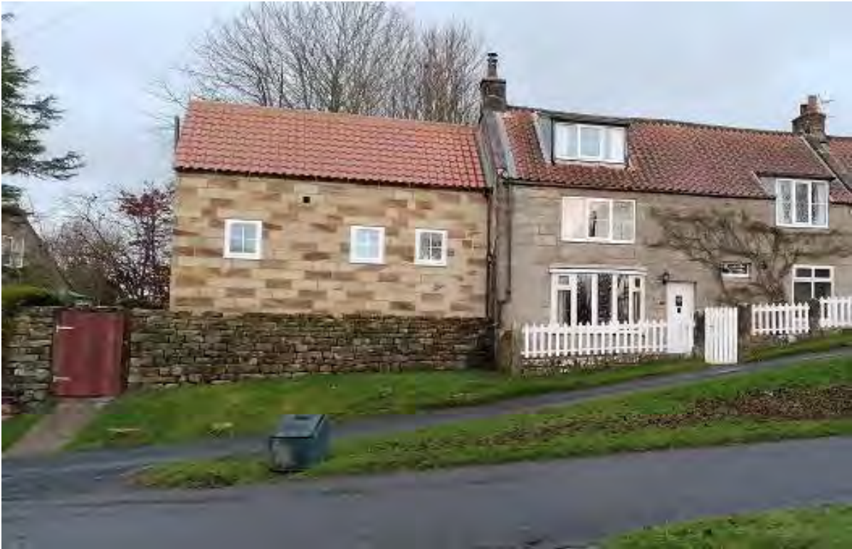
Photo showing front elevation of property with extension as constructed
