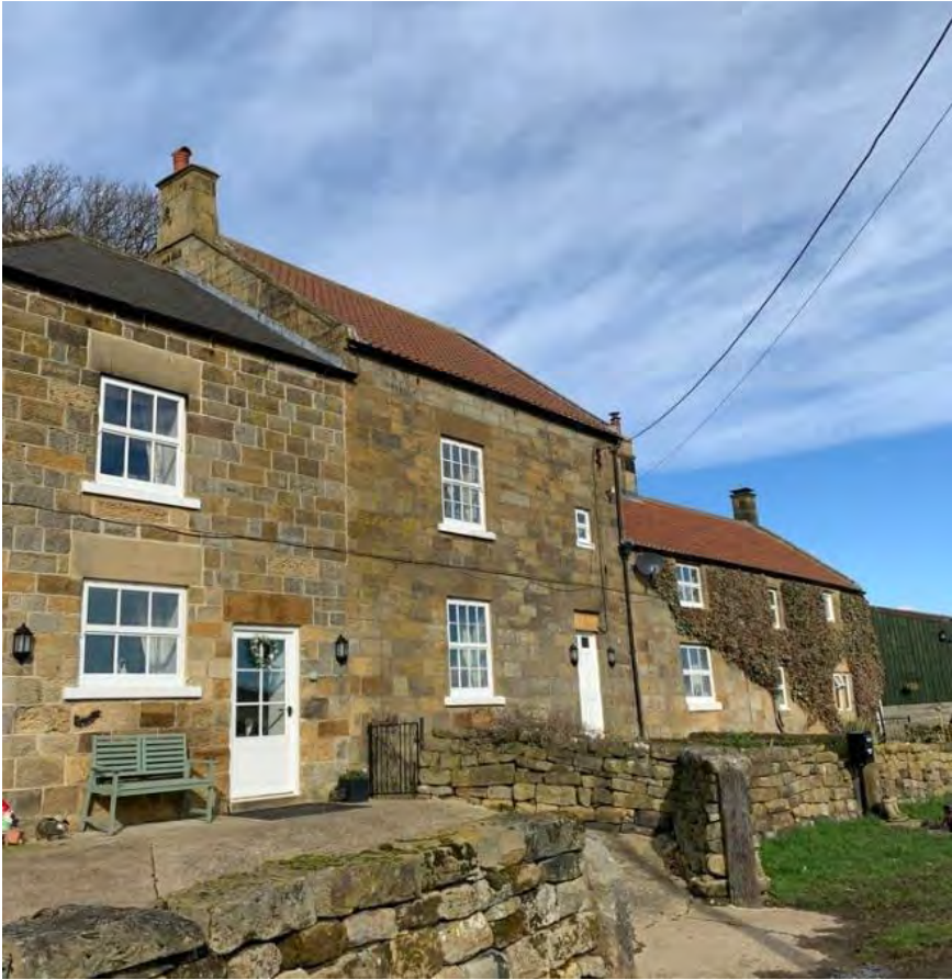
South elevation facing Dale
