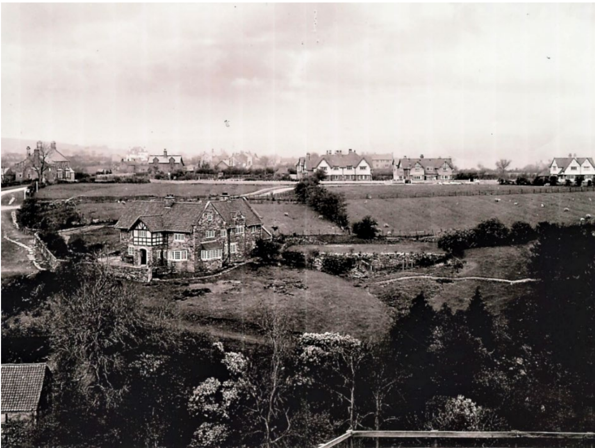
Figure 2 . Historic Aerial View of Goathland (the Goathland Hotel is in the background)
