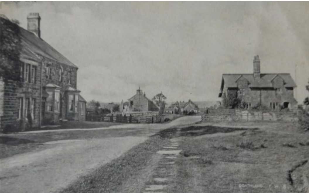
Figure 5 Bank Top Cottage was a crossing keepers' cottage, for the railway which crossed the road at this point. On the left, the Goathland Hotel built 1877 (historic photo courtesy of Eileen Peirson)
