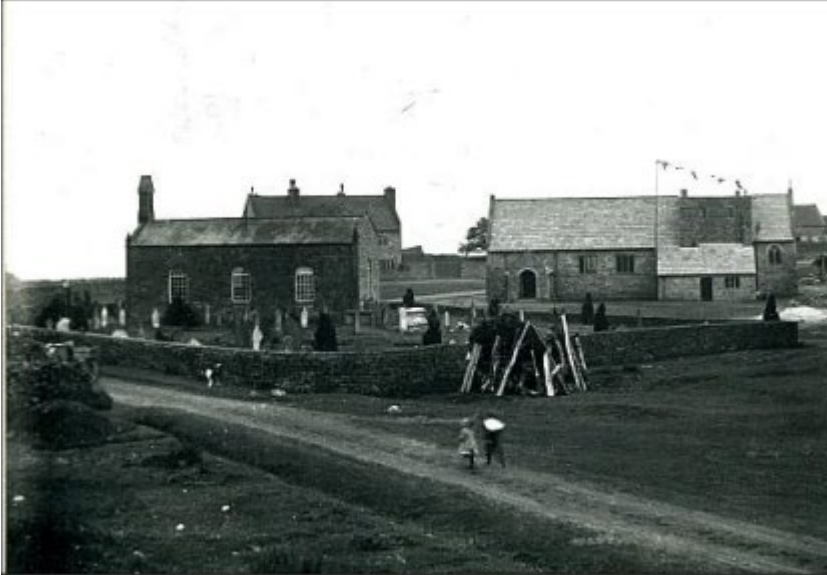
Figure 4 The present-day church under construction on the right and the 1821 church on the left, shortly to be demolished to provide stone for the church tower
