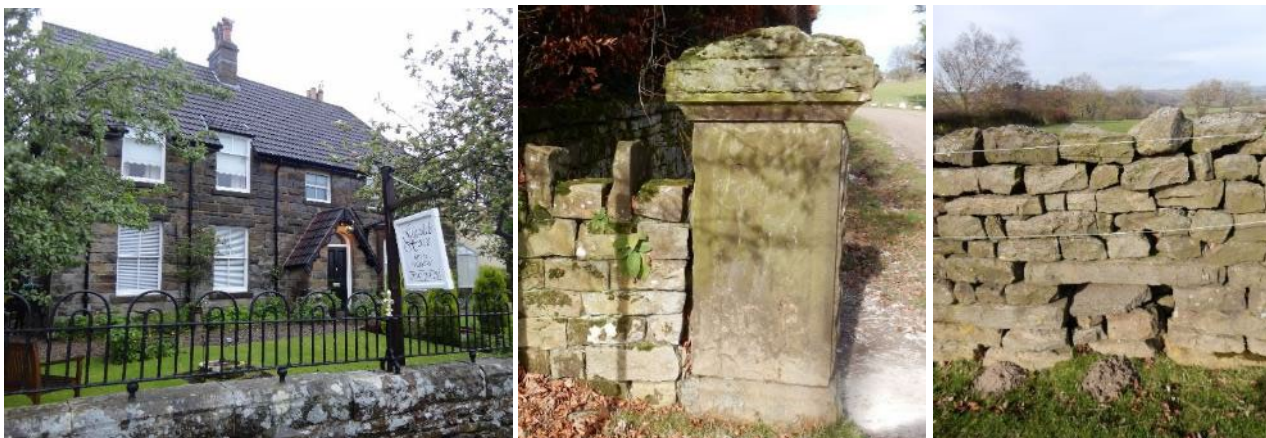
Figure 13, 14 & 15: A variety of boundary types. Left to right: a dry-stone wall with blocked sheep stoop; ornate iron garden railings on a dwarf stone wall; an ostentatious gate pier at an entrance drive
