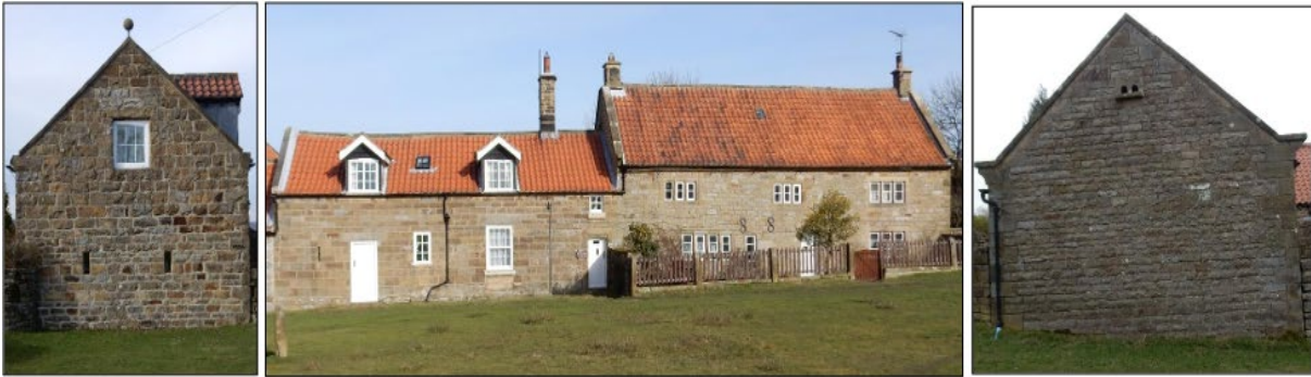
Figure 18. Agricultural architectural features. Left: slit vent windows reflect earlier use for livestock. Centre: a 1740 rebuilding of an earlier cruck longhouse with cross passage. Right: dovecots survive in some gable ends
