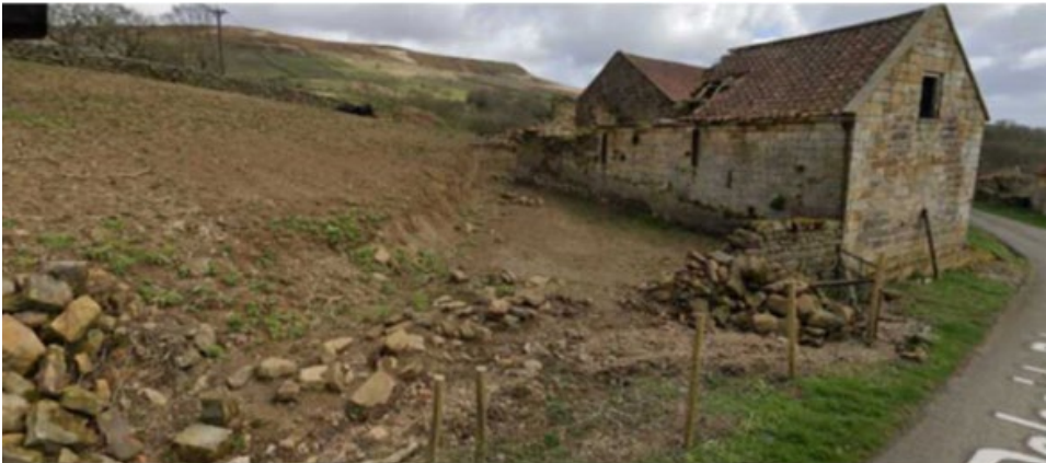
Photographs showing building condition prior to re-building works (Google Streetview, 2024).
