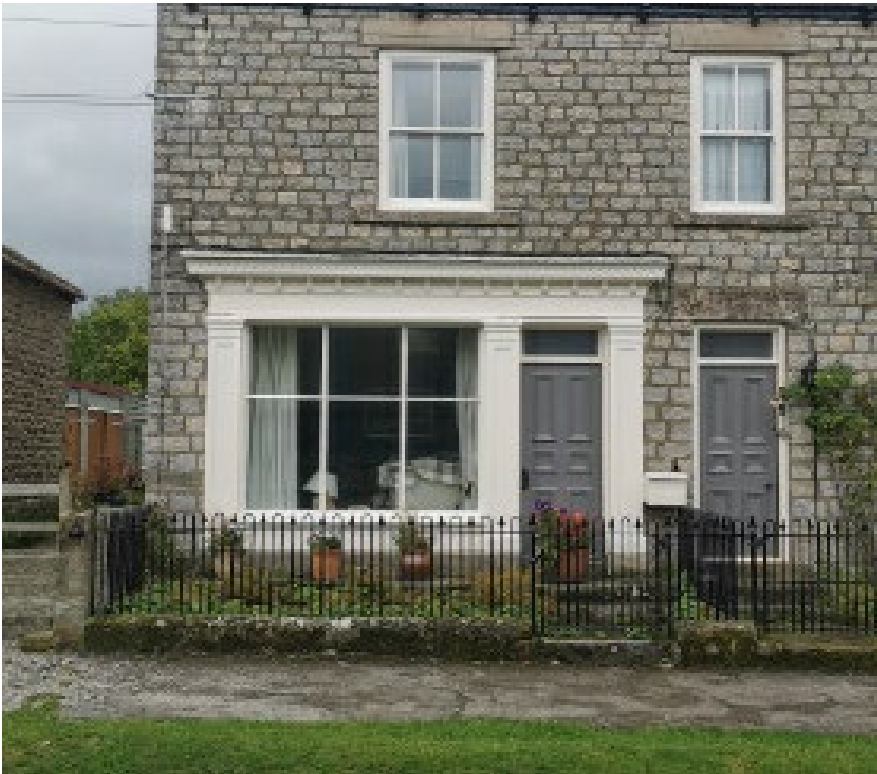
Figure 17 The only shop front in the village
