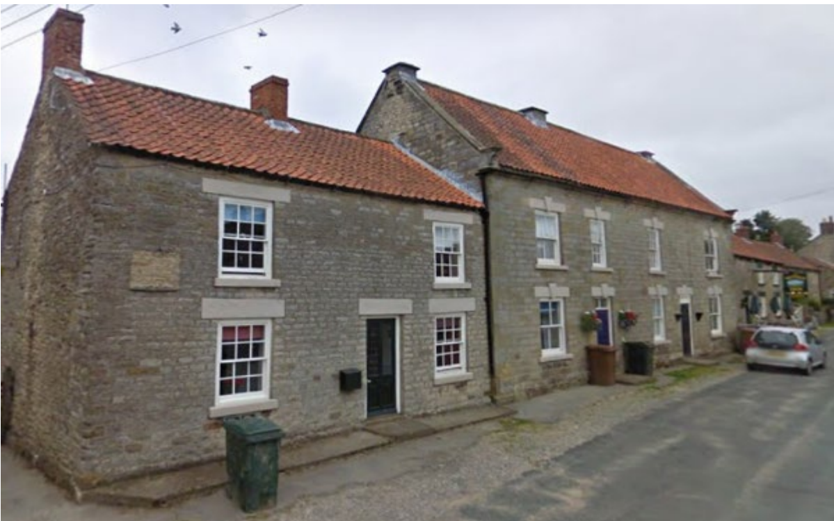
Figure 8 The need for off street parking is seeing the eroding of the grass verges as cars use them to park on
