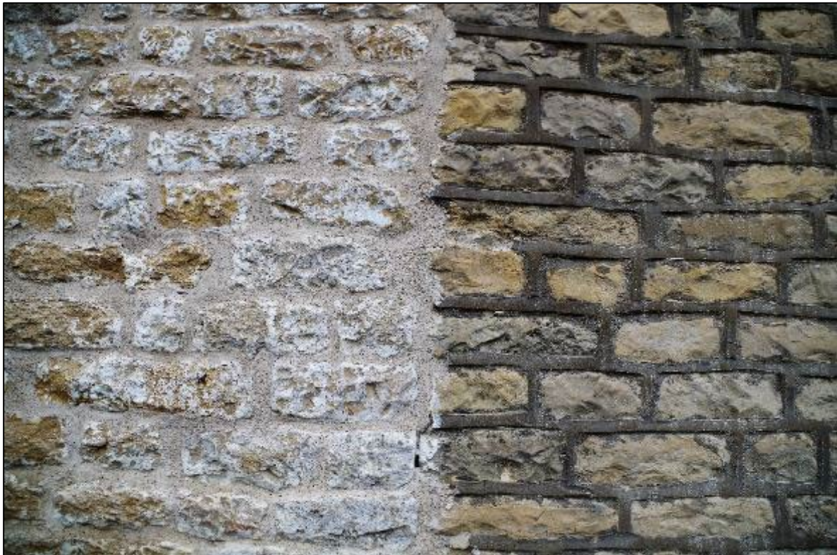
Figure 47: Different ownership has resulted in different approaches to pointing. The ribbon pointing on the right with cement will damage the stonework over time.
