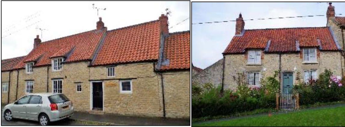
Figure 50 & 51: Cruck constructed houses at Cruck Cottage and Westfield Cottage
