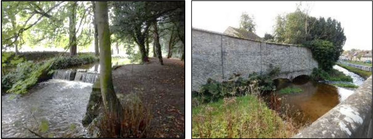
Figure 22 - 23 Left: The beck divides in the village centre; one half runs through the once private landscaped grounds of Thornton Hall and the other runs through the village. Right: The beck was diverted into two parts at Thornton Bridge with a private circuit around Thornton Hall furnished and another running parallel but outside the Hall grounds and along the High Street.
