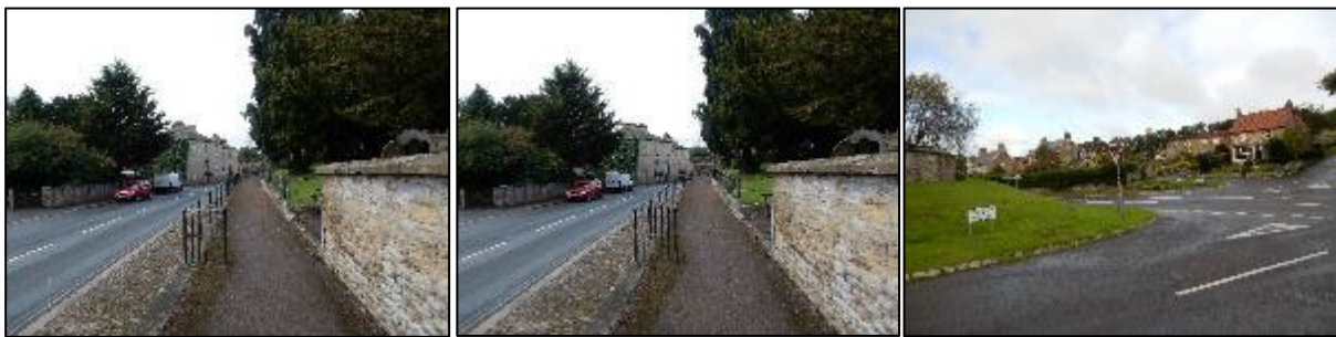
Figure 27, 28 & 29: The use of tarmac and painted traffic control lines particularly in the east end of the village has had an urbanising effect. This is softened by grass verges, stone steps, and a band of cobbles near the churchyard which narrow the road.
