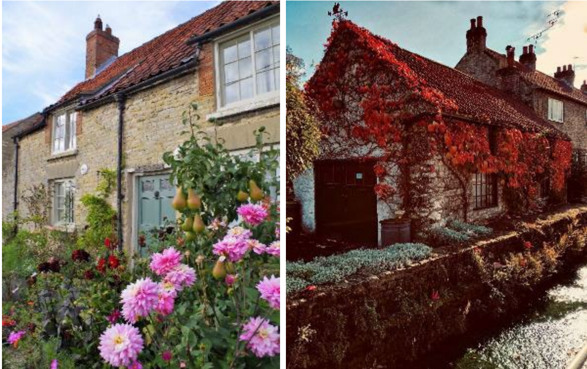
Figure 2: Left - Sandstone cottages under a red pantile roof, notice the Yorkshire Sliding Sash windows. Figure 3: Right – the village comes into its own in the autumn, with a mass of red Virginia creeper climbing up cottages (image by ayorkshirecurl)
