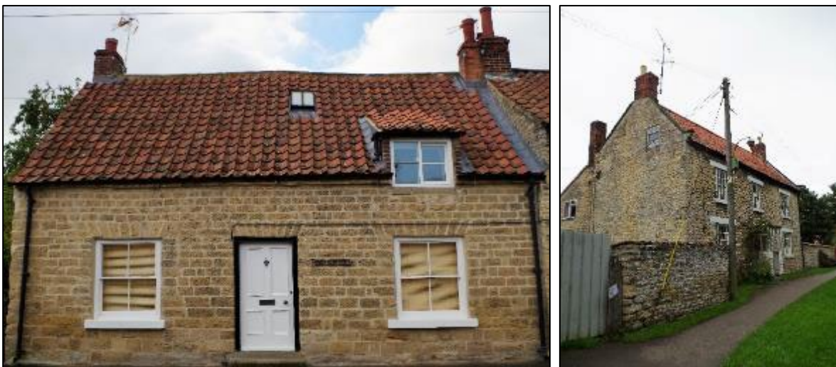
Figure 52, 53, 54 & 55: Typical examples of 18th century houses. Top Left: 18th century Rockingham House with symmetrical frontage and roof with pantiles, water tabling and
