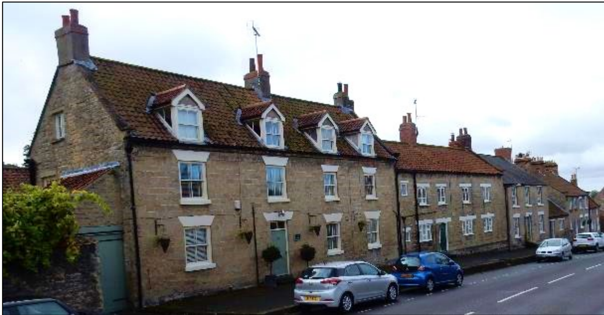
Figure 48: Red pantile roofing is the predominant roofing material and has replaced thatch since the mid-18th century. There are few examples of slate in the village.
