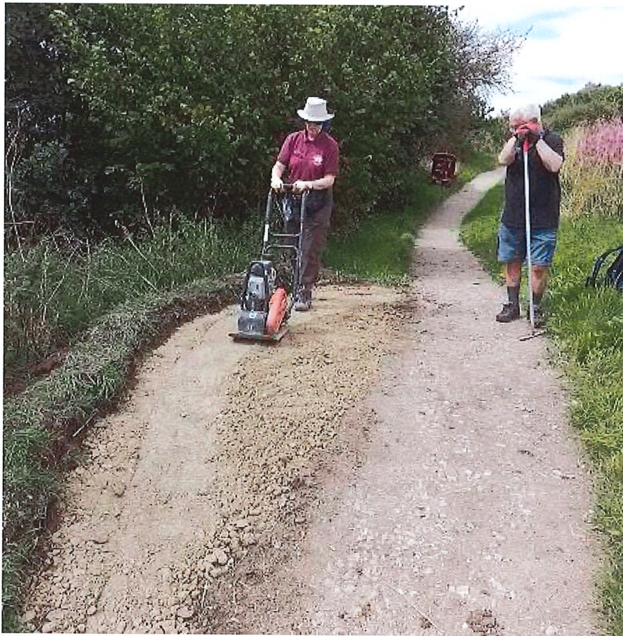
Constructing tramper layby August 2023
