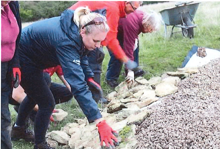
Securing the liner and reinforcing the bank - photo credit James Metcalfe
