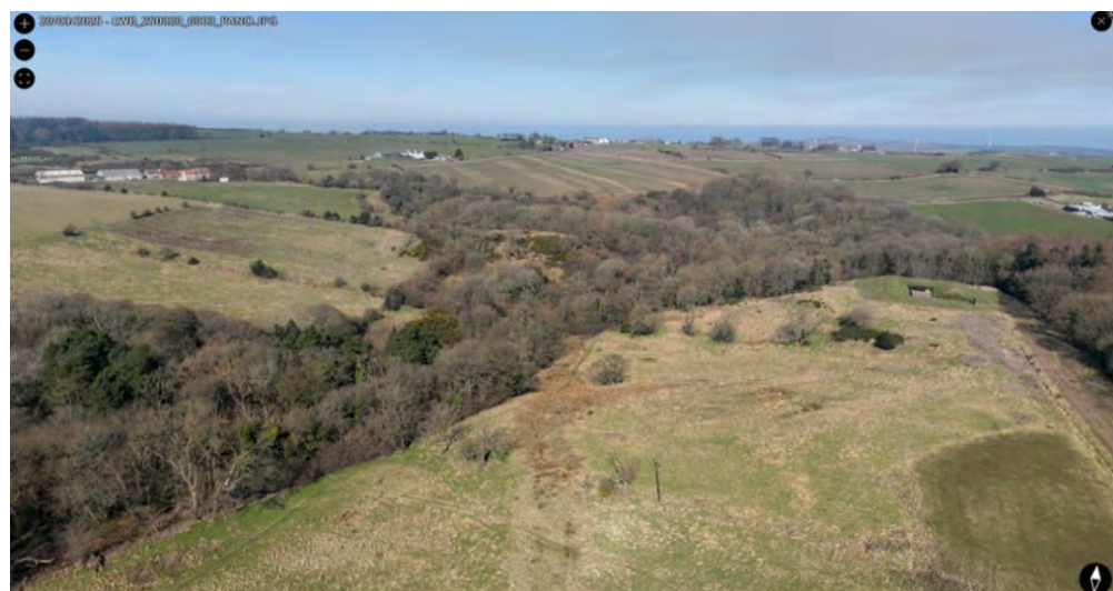
Plate 10: Lockwood Beck – Pre-construction (top) and 2025 (bottom)
