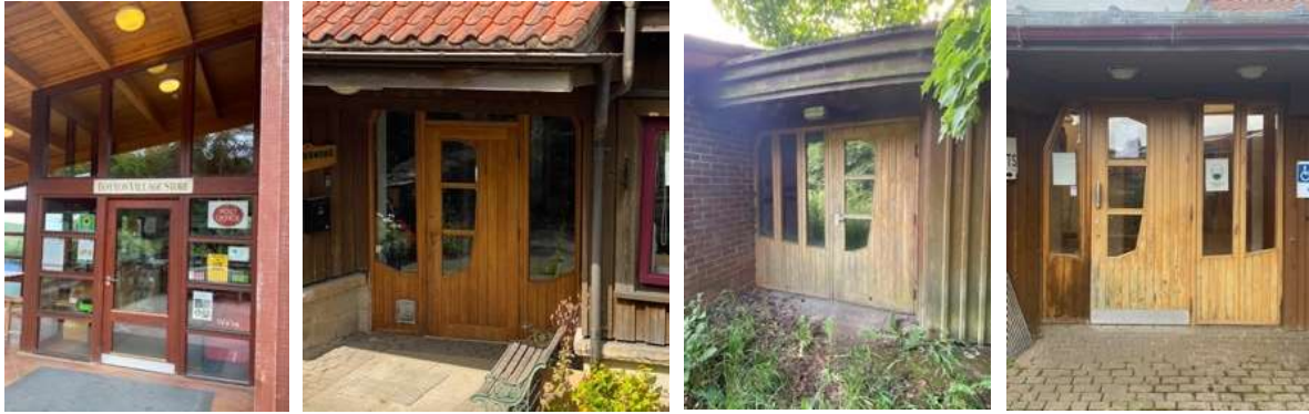
Doors at Village Shop, Lusmore, Ashwood and Stables
