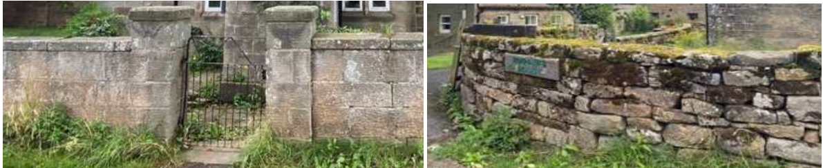
Formal mortared wall at Lodge and dry stone at Rodger's House
