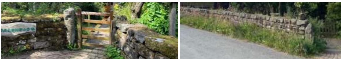
Dry stone walls at Dalehead and Lusmore
