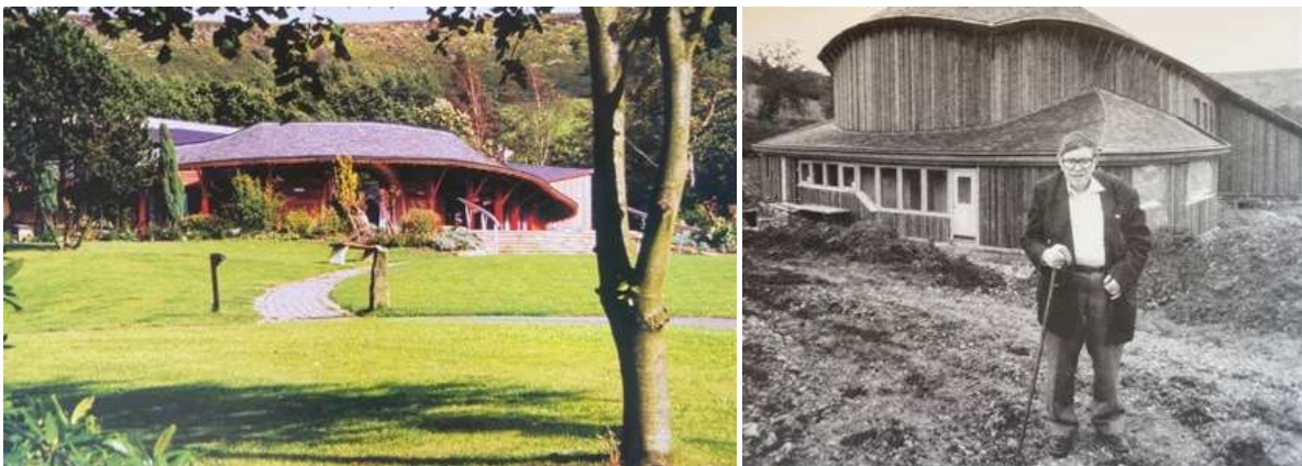
The remodelled Community Centre and the Chapel 1998
