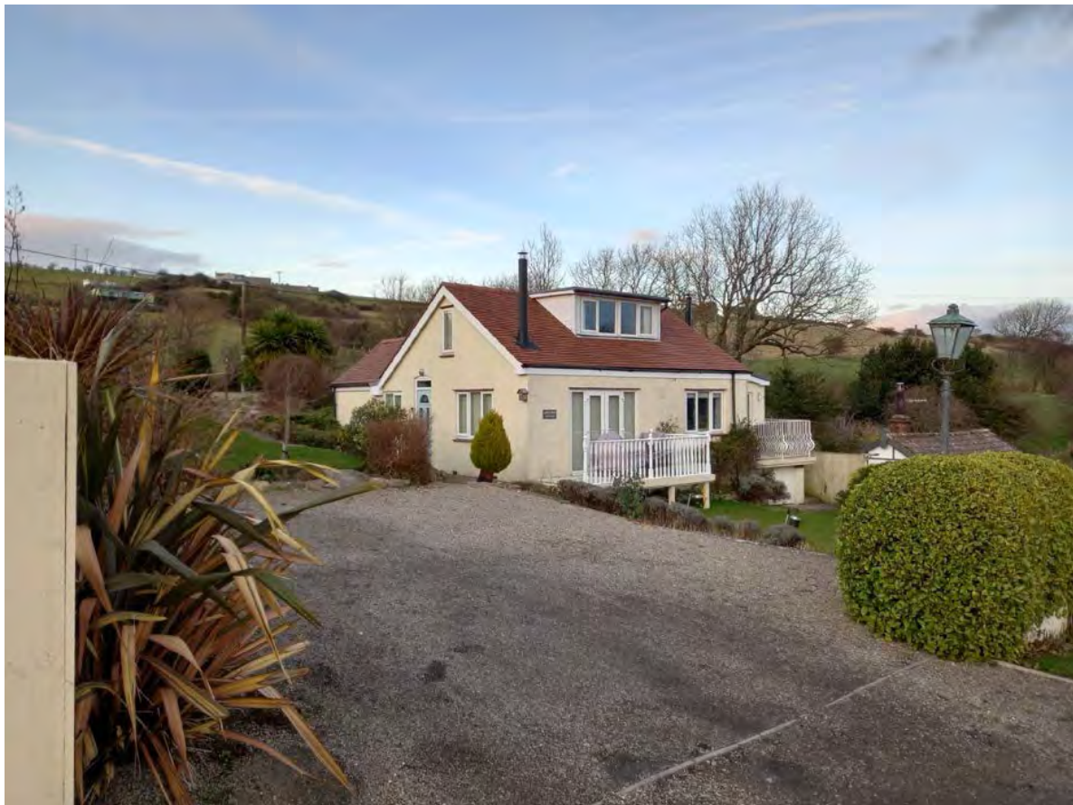
Photo showing front elevation of the property with the dormer and raised decking areas to be replaced
