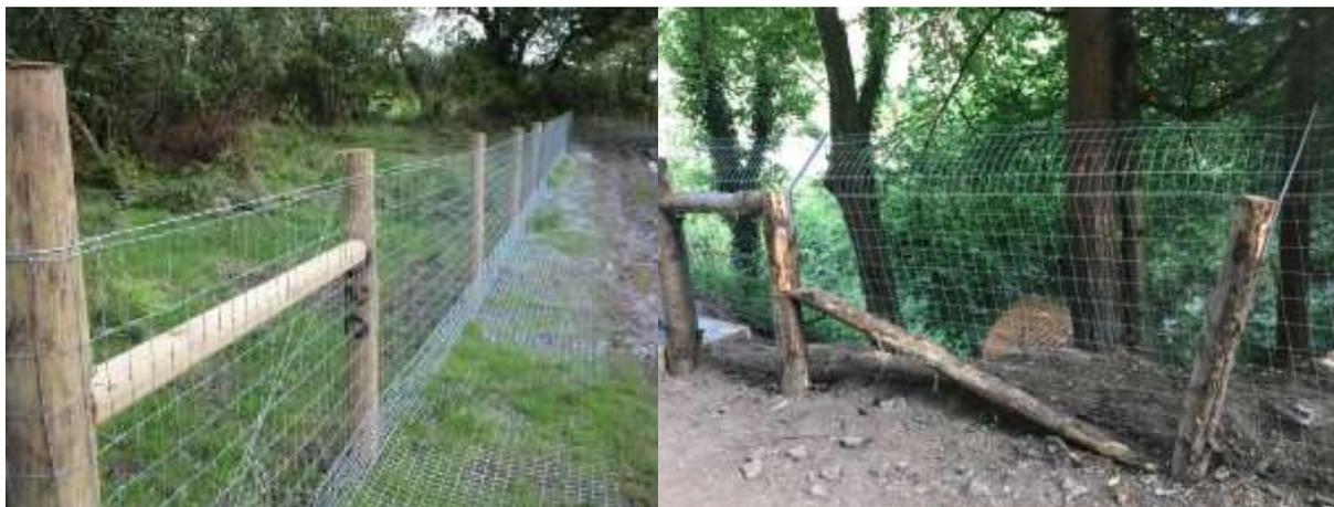
**Fig.6** Examples of beaver proof fencing to discourage digging, climbing and
