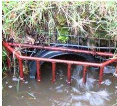
**Fig. 8** Metal grilles to protect culvert. Robust bank meshing and heavy set grille which is fixed to bank side and stream bank to withstand beaver digging around inflow.
