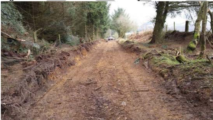
Figure 11: and after vegetation clearance, re-profiling and drainage 2017
