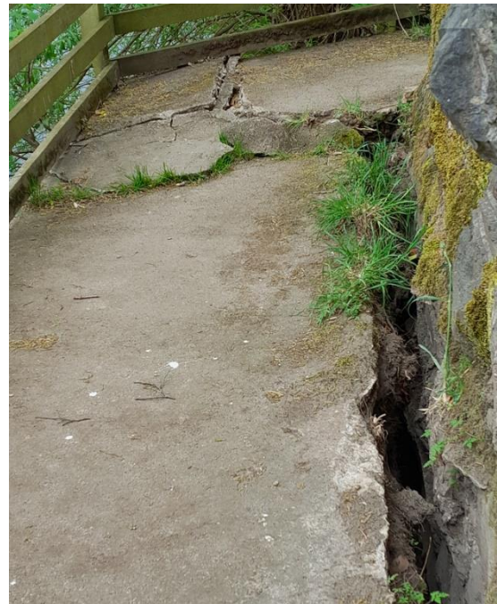
Photos showing the slumping and movement of the revetment, and subsequent collapse.
