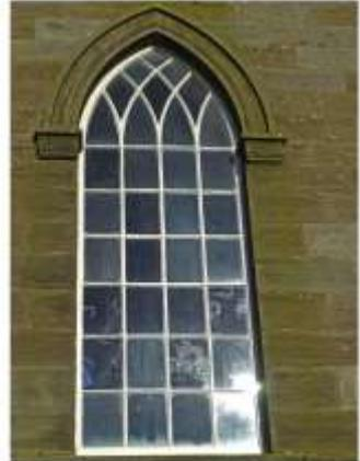
Windows repaired and re-decorated. Fingerprints indicate glass replacement (these were removed before the contractor finished). Traditional burnt sand mastic has been used between the frame and masonry reveal.
