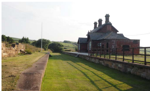
Fig.76 Former station and platforms at Kettlewell
