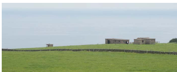
Fig.77 WWII coastal Radar station at Ravenscar
