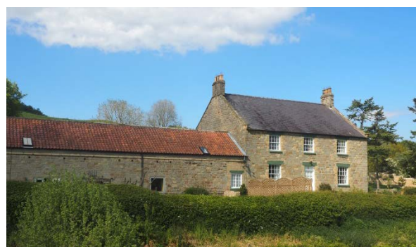
Fig.108 Traditional farmhouse at Mowthorpe Bridge
