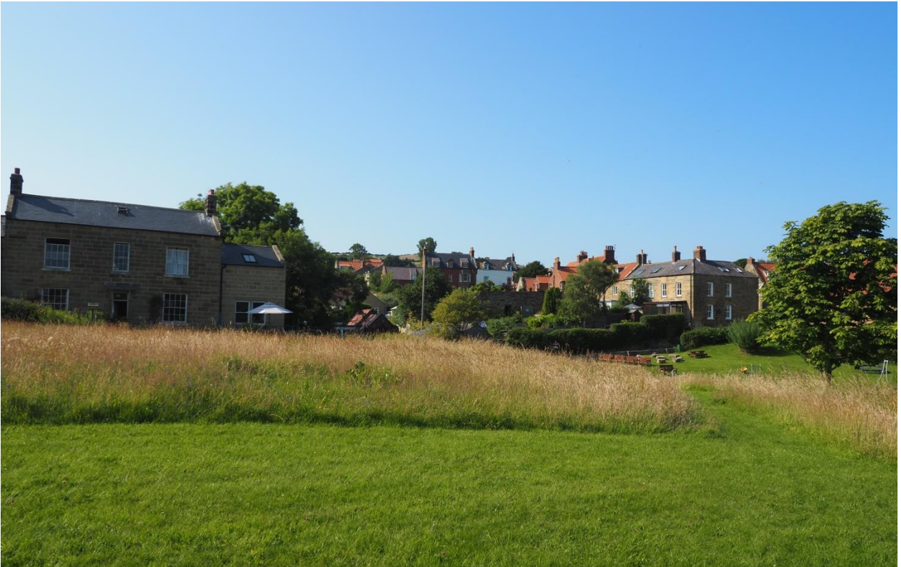
View from the Green, looking north. The stone houses are within the historic core and Conservation Area
