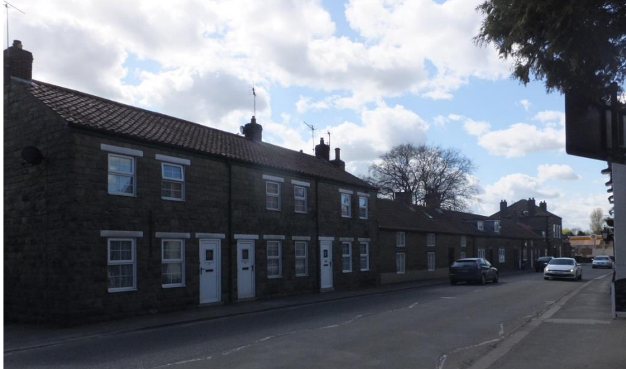
Photo 37: Traditional buildings with modern uPVC windows, doors and dormers
