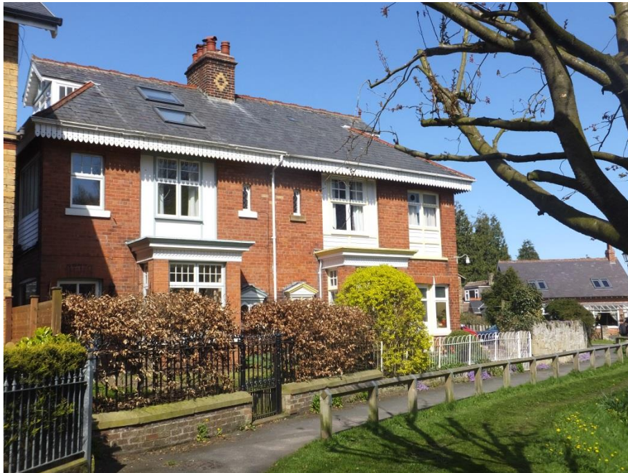
Photo 26: C20 buildings south end of Hall Garth Lane
