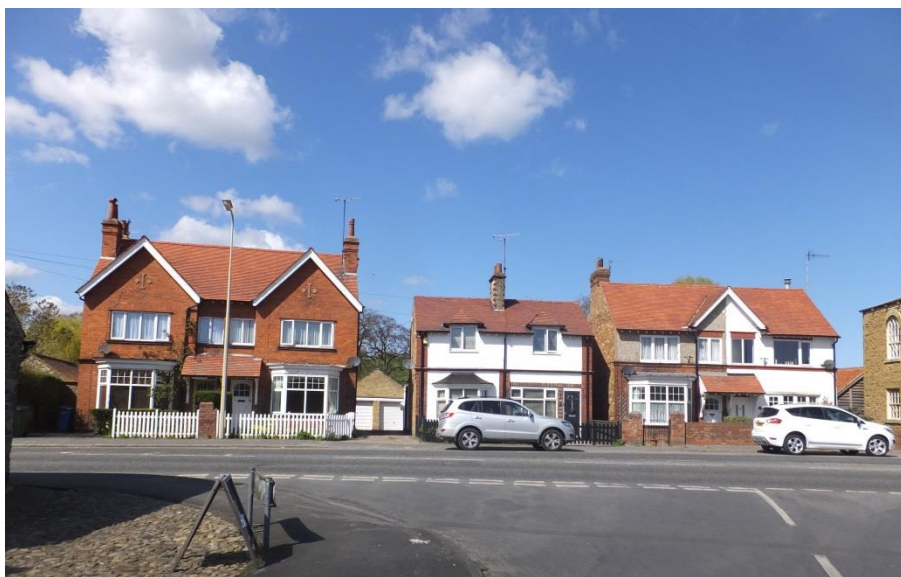
Photo 24: View of C20 buildings on Main Street
