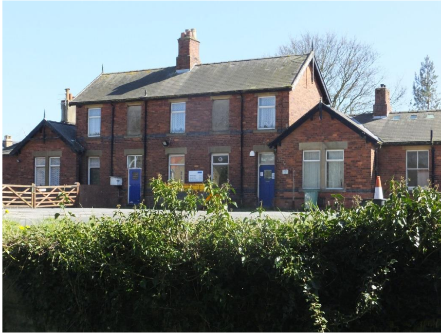
Photo 14: View of the former railway station
