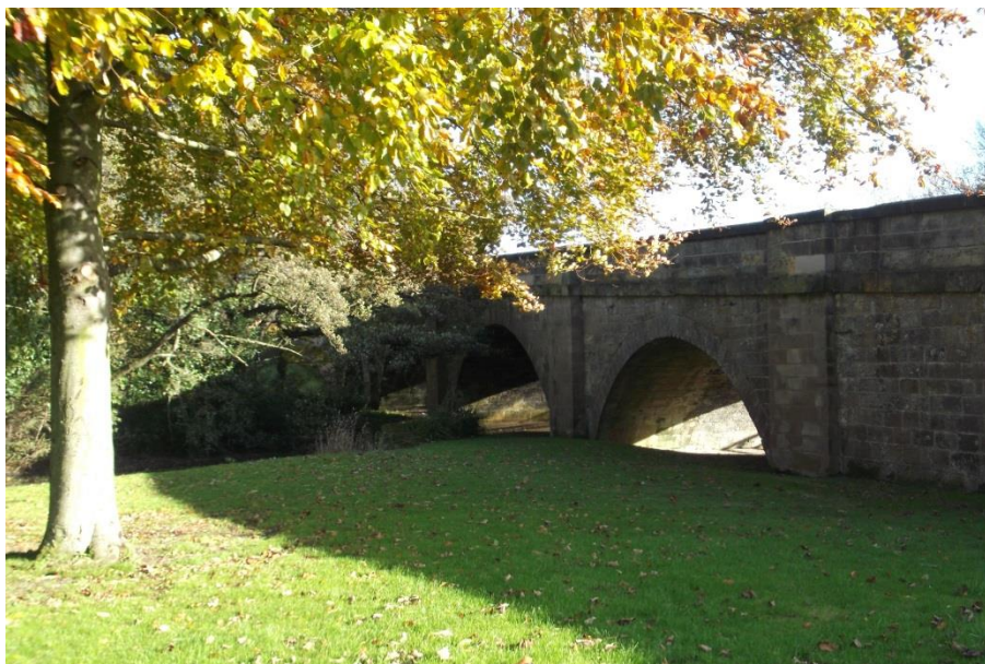
Photo 23: View of the Bridge
