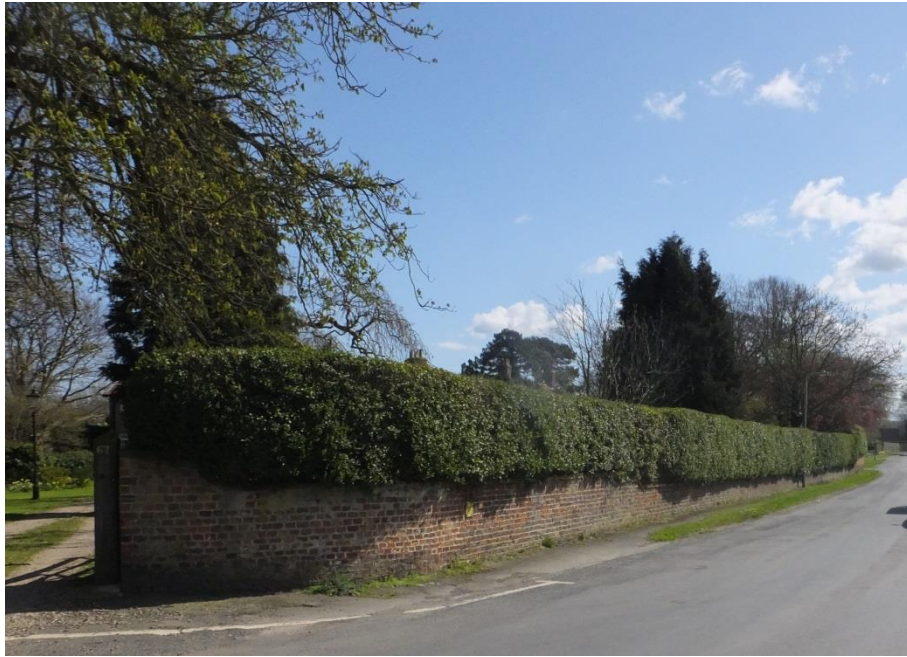
Photo 27: Boundary wall along Hall Garth Lane
