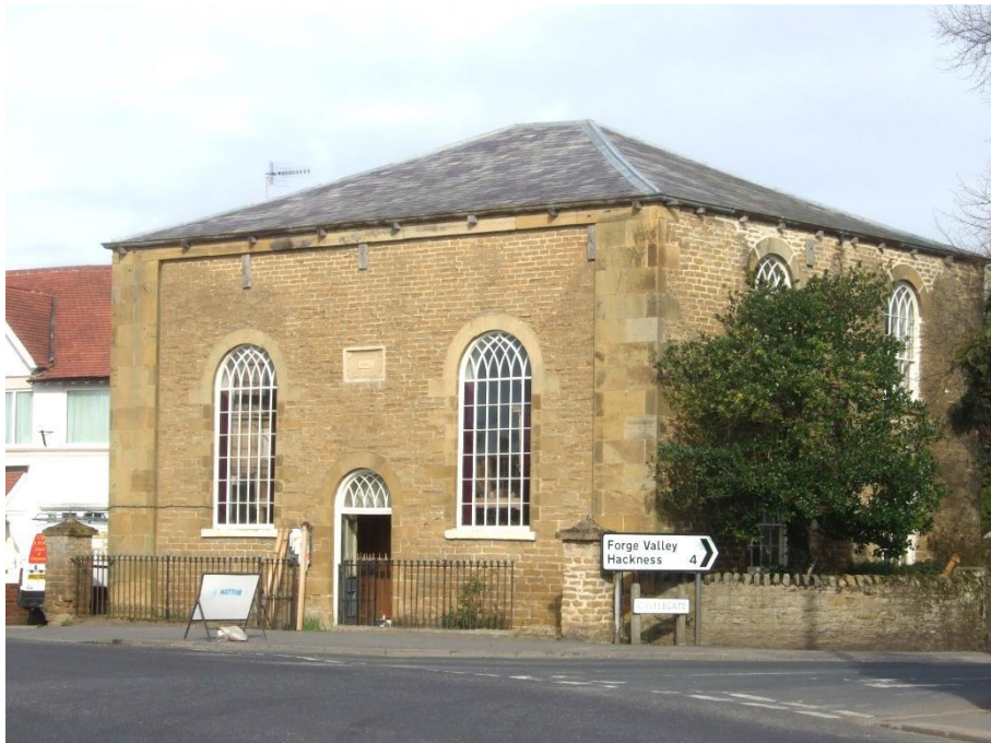
Photo 30: View of the former Ebenezer Chapel
