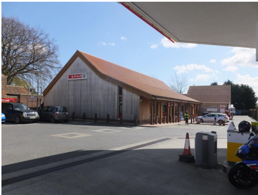
Photo 12: View of the Petrol Filling Station
