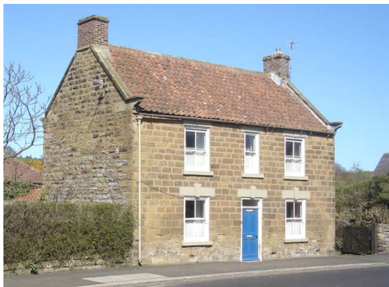
Typical materials, local details and storey heights
