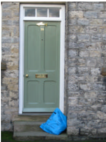
Photograph 12: Vernacular Door Detail
