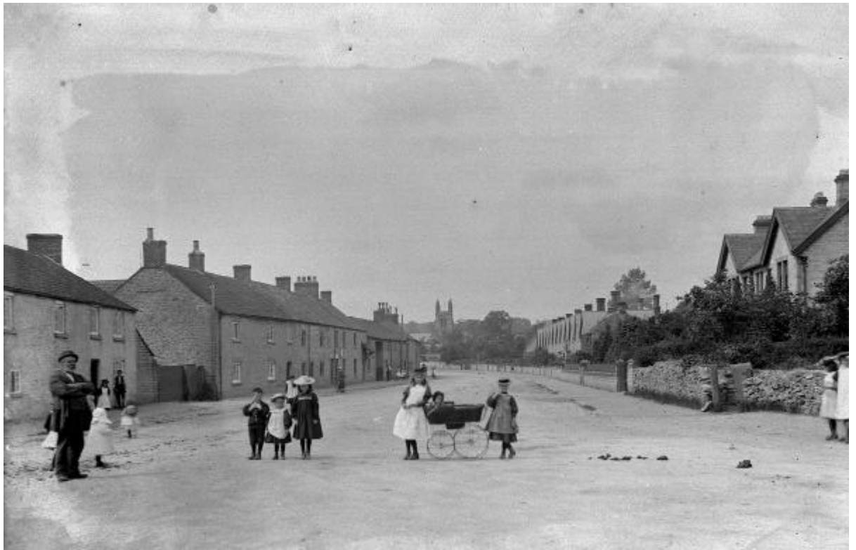
View west along Bondgate
