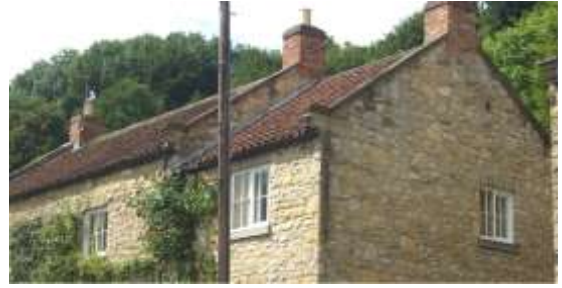
Stone water-tabling, kneelers and cast iron rainwater goods
