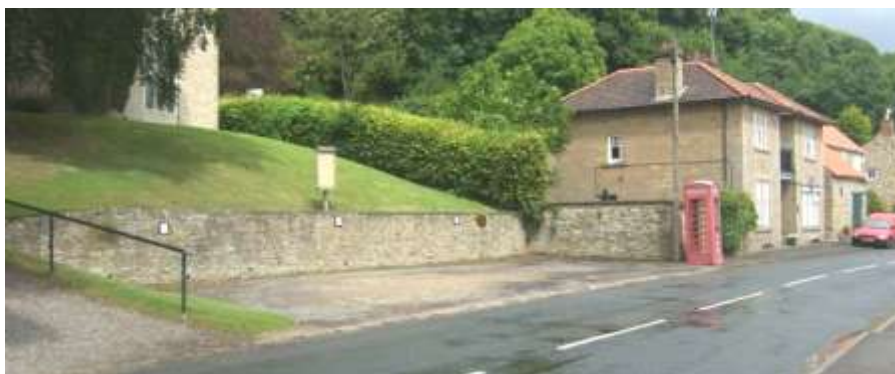
Loss of traditional boundaries and areas of hard standing can be detrimental to the street scene
