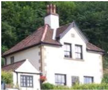
Crag Cottage, Main Street: central chimney stack
