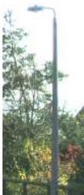
Concrete street light in Manor Close
