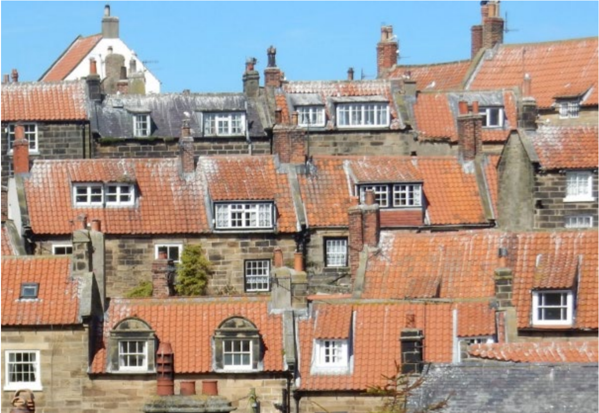
Figure 47. A roovescape view of Robin Hood's Bay showing the different styles of dormers.
