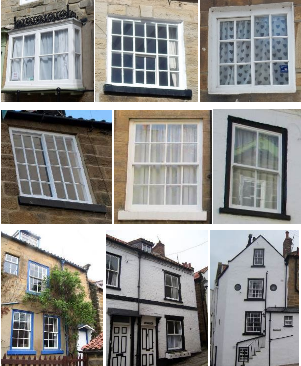
Figures 38 – 46. A selection of the varying window designs and paint colours found in Robin Hood's Bay.
