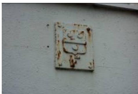
Image 5.39: Cast iron fire hydrant
