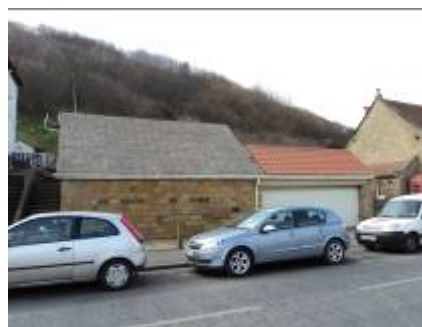
Image 5.32: Garage / storage building
