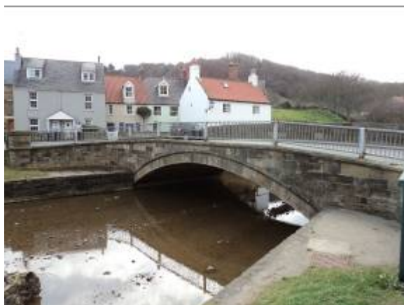
Image 5.23: East Row bridge
