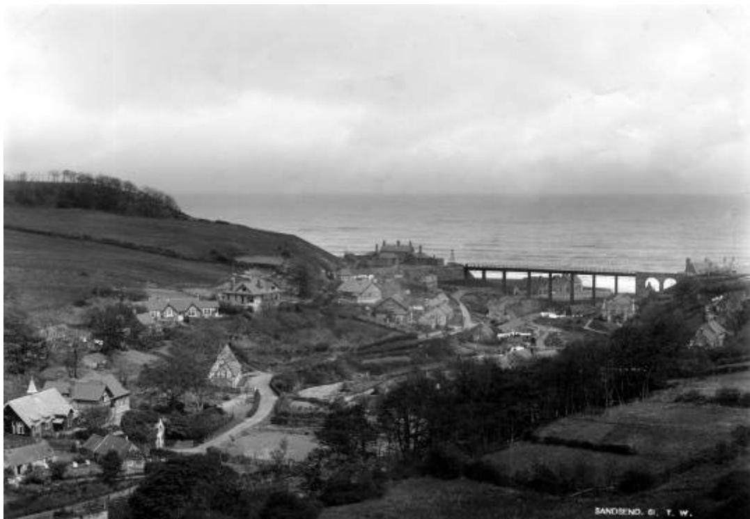
E.4 – Sandsend Beck and viaduct
