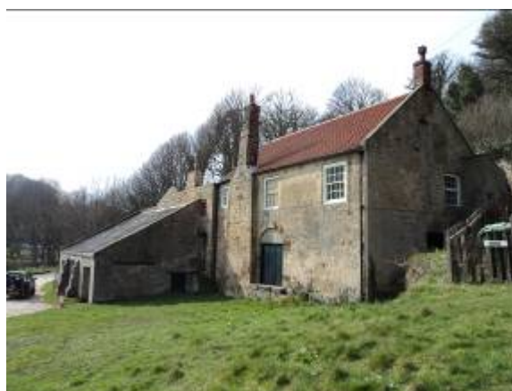
Image 5.28: Mill Cottage with 'Roman Cement' Mill attached
