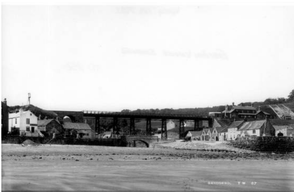
E.16 – Sandsend viaduct and alum house yard
