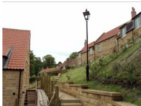
Image 5.11: Street lamp in new development
