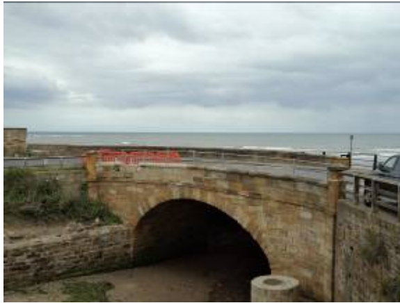
Figure 5.12: Sandsend Beck bridge
