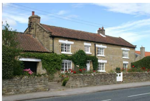
Holly Bank the combination of stone, pantile parapetted gable ends and dry stone boundary wall characterise the area
