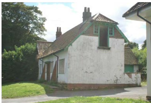
Vacant building on Hackness Road
