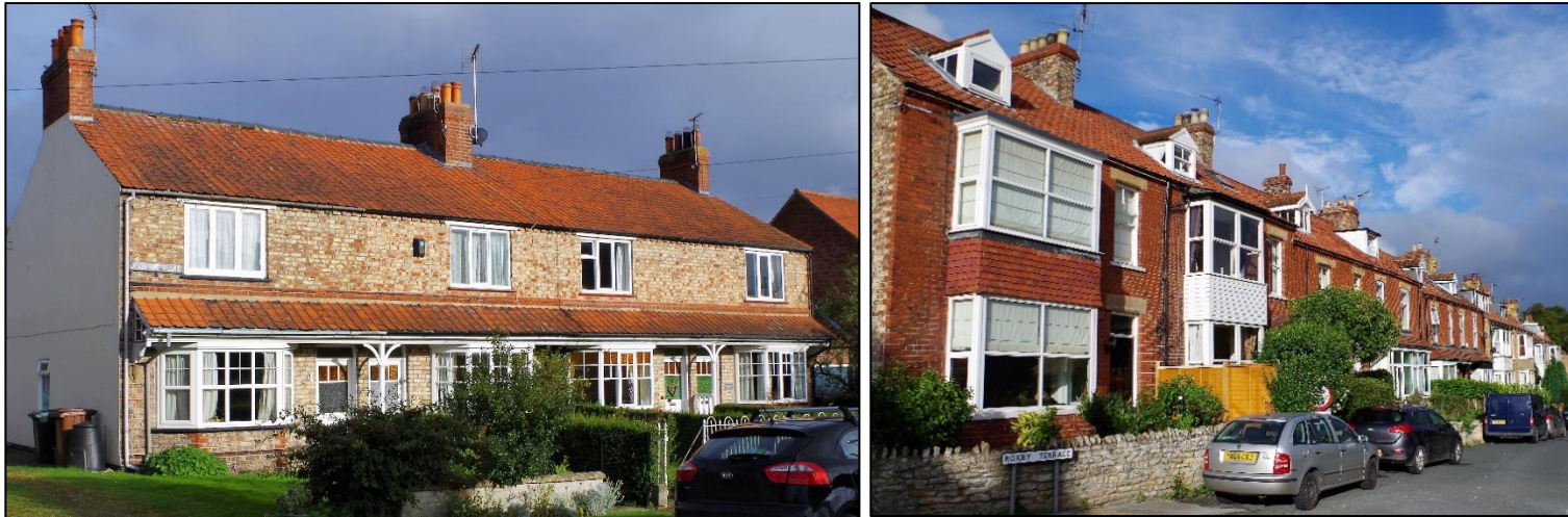
Plate 23. Jessamine Villas and Roxby Terrace represent early 20 th century building stock which tends to suffer from not being old enough to list and so traditional features are lost. However both rows have good survival of traditional timber doors and porches and stained glass windows.
