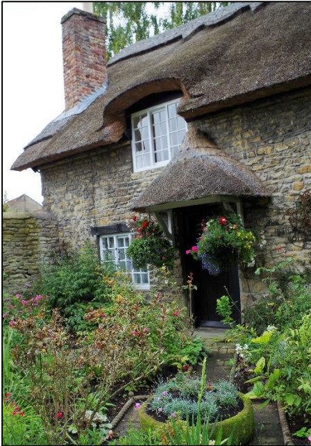
Plate 18. Thatch was once commonplace and is now restricted to Beck Isle Cottage
