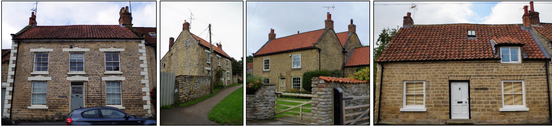
Plate 20. Typical examples of 18 th century houses. Left: The late 18 th century Rockingham House with symmetrical frontage and roof with pantiles, water tabling and kneelers. Centre left: The use of small eaves windows in 18 th century gables is also a common feature and the former steep pitch suggests that this building was once thatched. The catslide roof to the rear is a common method of extending such houses. Centre right: Brook Farmhouse has similar symmetrical features, pantiles, water tabling and kneelers but is a double pile house, typical of higher status houses and also seen at High Hall. Right: an altered 18 th century cottage with later windows and door.
