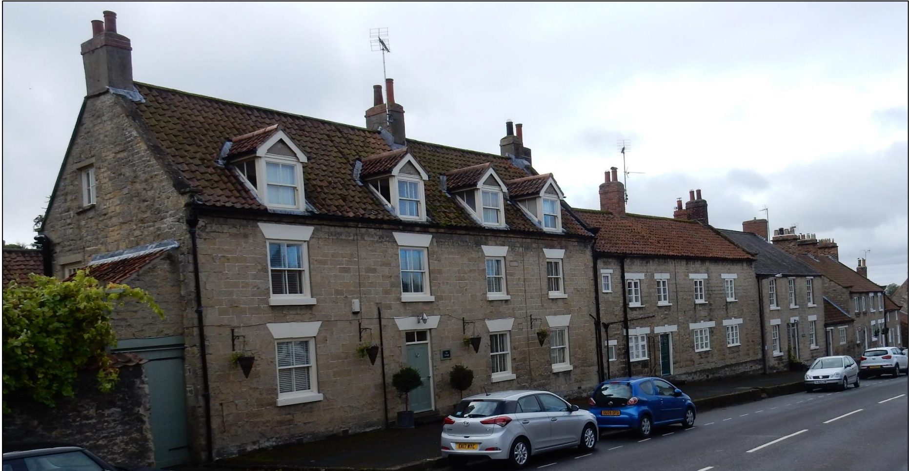
Plate 17. Red pantile roofing is the predominant roofing material and has replaced thatch since the mid 18 th century. Some other roofing materials have been used since the 19 th and 20 th centuries but are not characteristic. There is some stone water tabling and use of kneelers on 18 th century buildings, but the majority are without these features.
