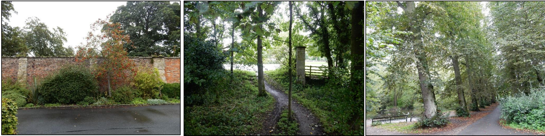
Plate 7. Left: The brick and stone kitchen garden walls, now used as a car park, but with perimeter planting to reflect a continuing horticultural use. Centre: The end of the kitchen garden wall is dressed and suggests that the garden was never fully enclosed but open to the south. Right: A lime avenue linking the kitchen garden to Maltongate.
