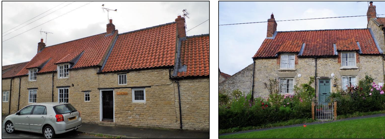
Plate 19. Cruck constructed houses at Cruck Cottage and Westfield Cottage
