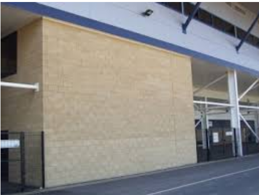
Figure 4.5 Fair faced block work
