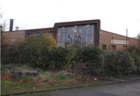
Figure 4.7 Use glazing bars and architectural metalwork break down the scale of the building
