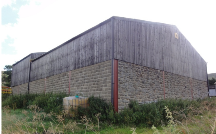
The use of stone helps to link the building to the more traditional buildings on the farm. A higher standard of material has been used on the most prominent elevation.
