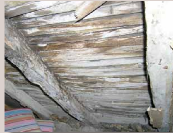
Lath parging to pantile roof in South End.
