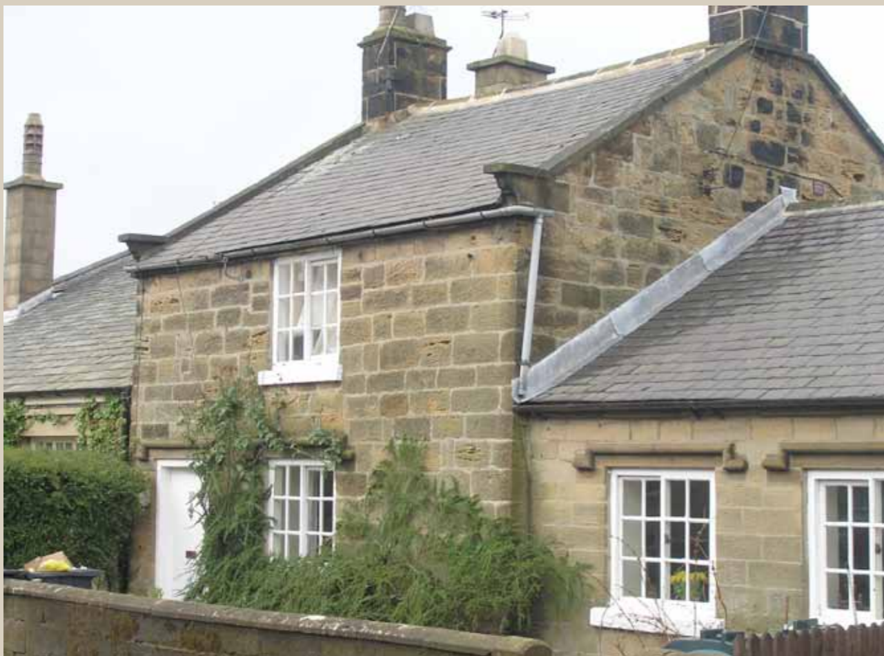
Yorkshire sash sliding windows in cottages dating back to early C18th
