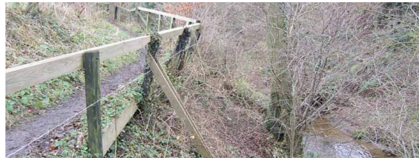
Dilapidated footpath between Thimbleby and Osmotherley
