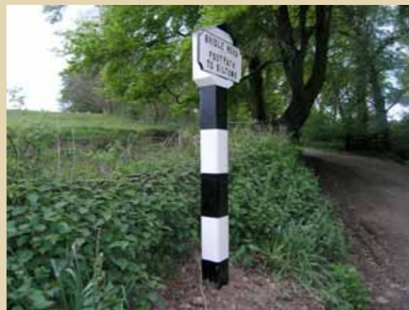
Restored timber sign. Both villages have timber lamp posts and telegraph poles from 1951, which have lasted without maintenance much longer than steel or plastic street furniture
