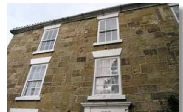
The Old Hall – with Jacobean windows outlined in the stonework beneath Georgian sash windows, yet with a hidden timber frame suggesting mediaeval construction.
