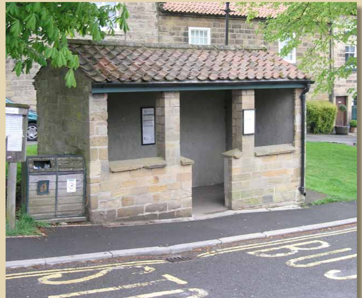
A good well-used bus shelter but with scope for minor improvement
