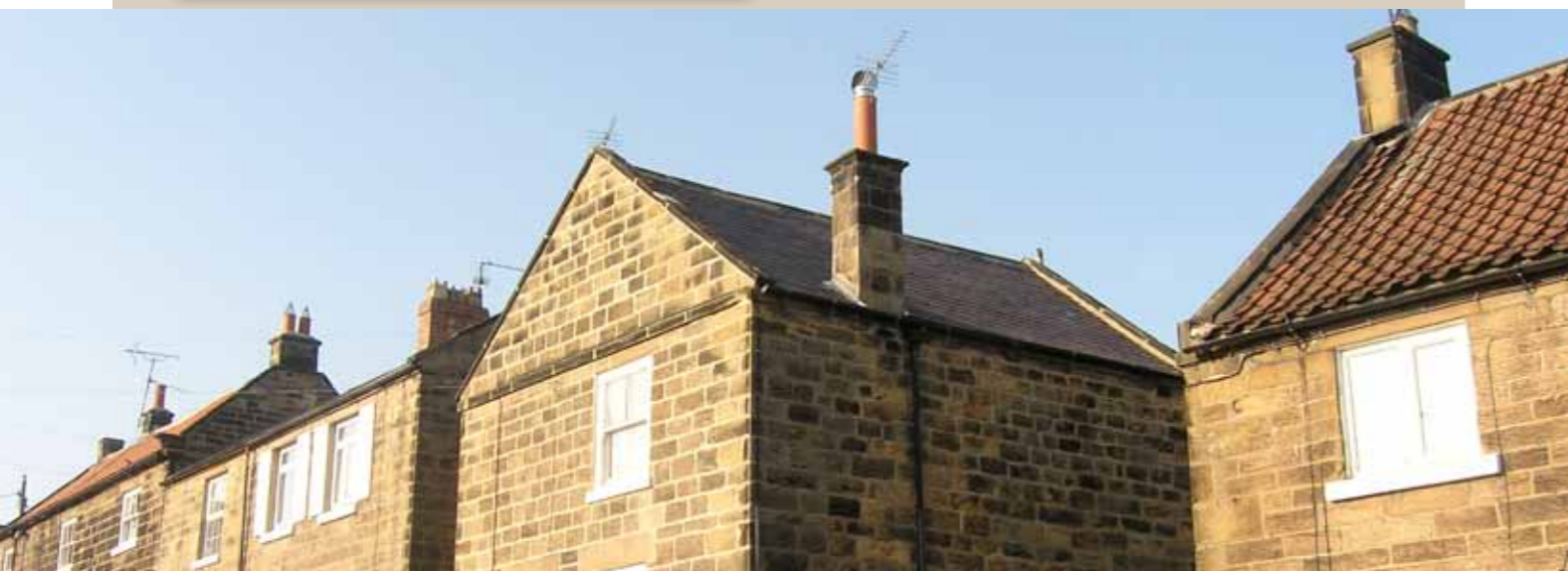
Variety of kneelers, string courses, roof cladding and orientation of chimney stacks
