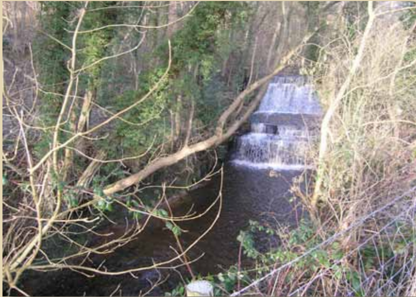
Two of many weirs on the Cod Beck used to power at least 7 mills or hydro-electric generators.
