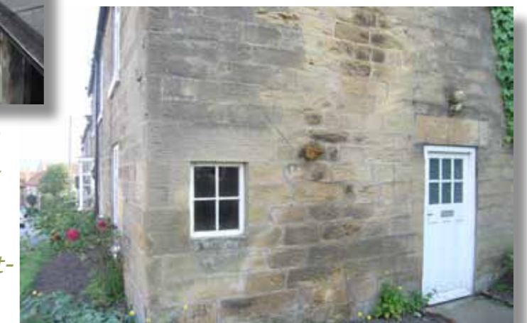
Above: Weavers window by the chimney flue.
