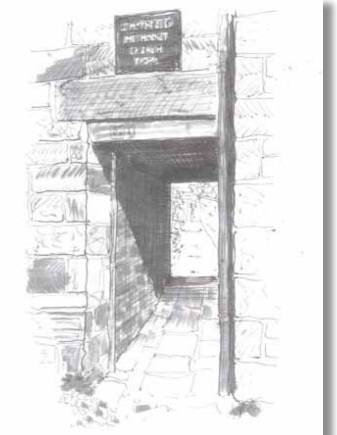
One of several timber lintels in Osmotherley drawn by the late Tony Lester
