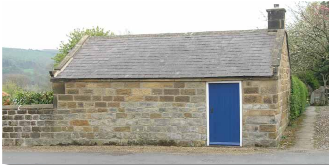
Outbuilding with chimney flue
