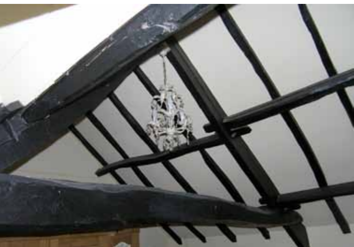
Above is an example of original timber framing
