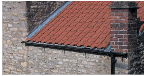
Black half-round plastic guttering is reminiscent of cast iron
