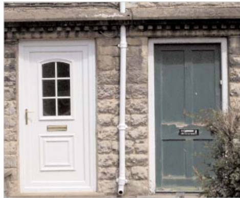
Modern uPVC (left) versus Traditional timber
