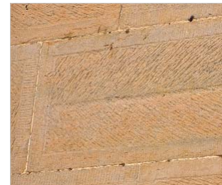
Ashlar stonework with fine lime-putty pointing
