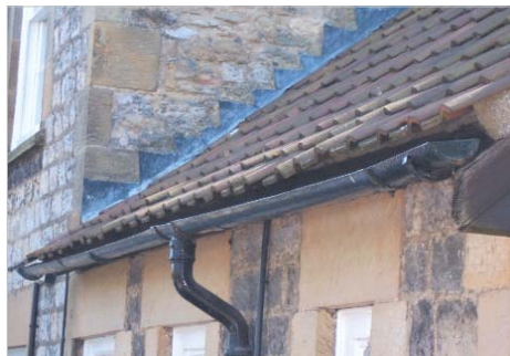
Half-round cast iron gutter (no fascia)
