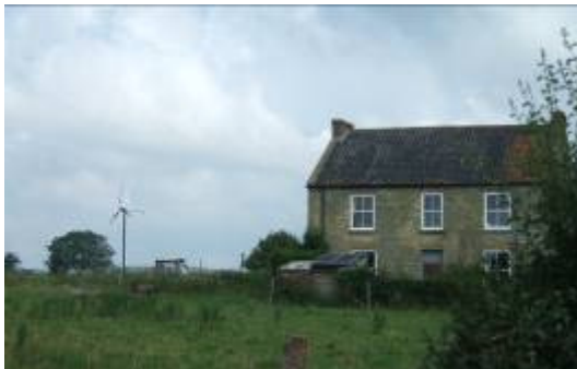
A wind turbine should be sited so that it relates well to the host building in terms of size and distance from the building(s), such as in this example.
