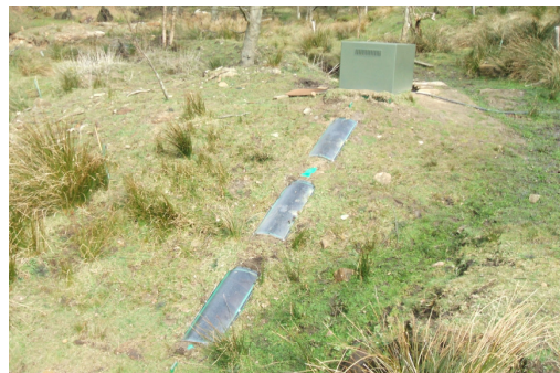
Pipelines can be located underground – in this example windows have been left so that the working turbine can be seen. . Painting the machinery housing green helps to conceal it.
