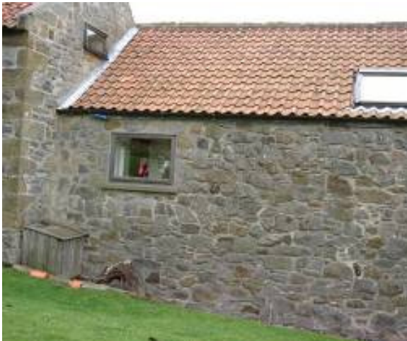
The pump (bottom left of picture) can be housed in an appropriately designed structure.
