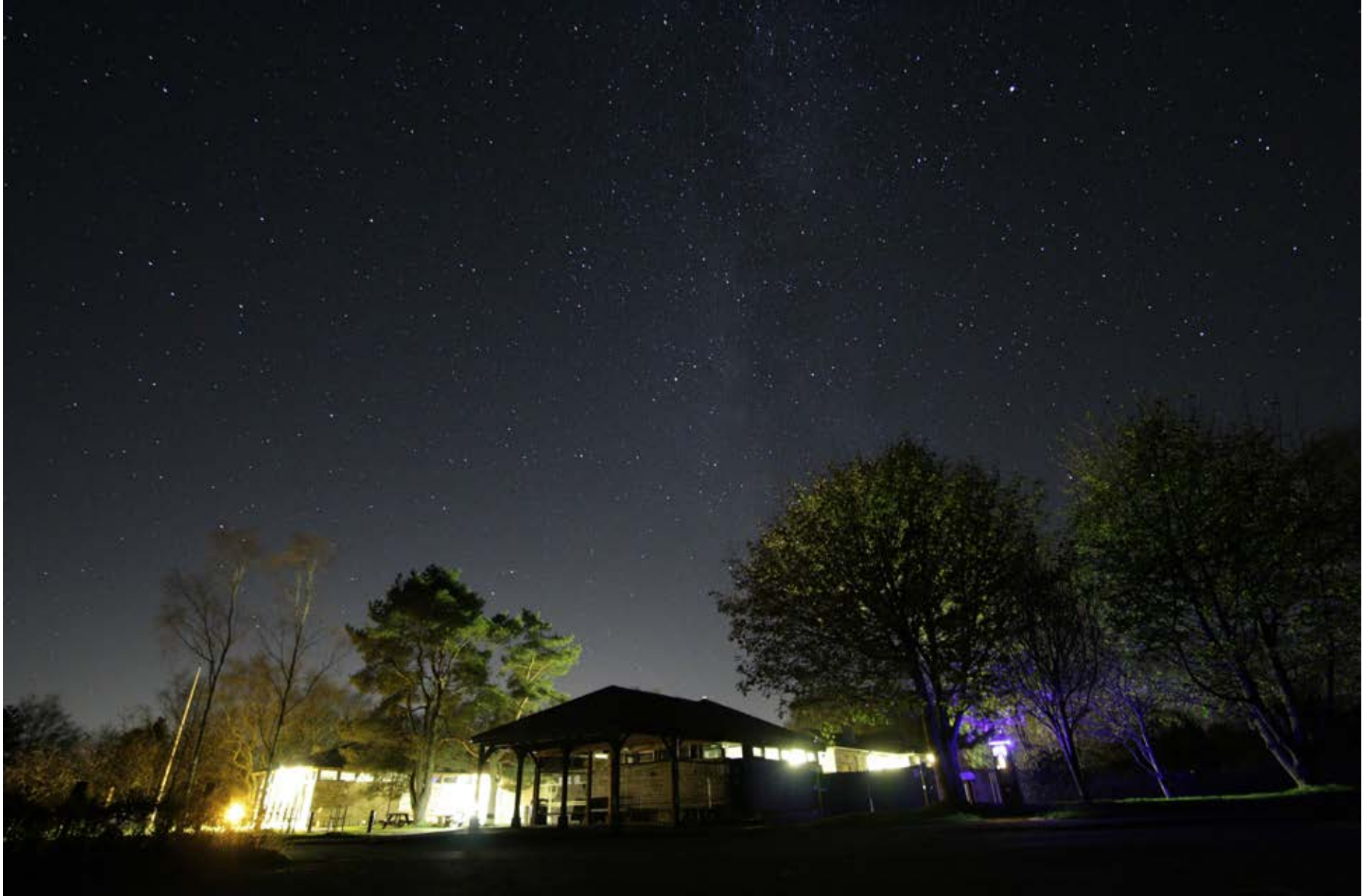
Sutton Bank National Park Centre at night, prior to work on dark sky friendly lighting commencing
