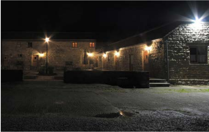
Rawcliffe House Farm – before
