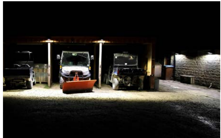
Cropton Forest Cabins – after, all lights on curfew or proximity sensor
